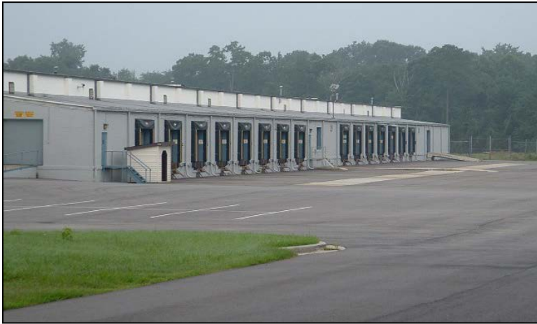
Figure P.4 Unloading Area of Warehouse.
