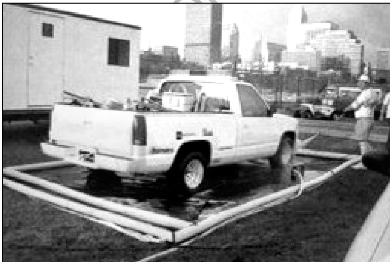
Figure P.3 Containment System Preventing Wash Water from Entering the Storm Drain.
