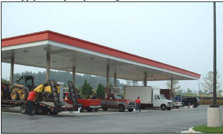
Figure P.2 Covered Retail Gas Operation Without Containment for Potential Spills.
