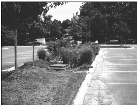
Figure 2: Parking Lot Island Turned Bioretention
