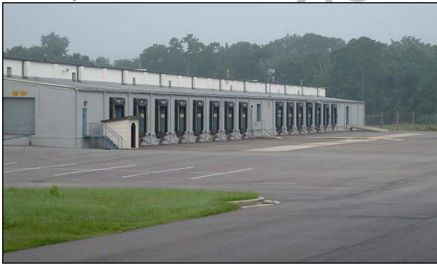
Figure P.4 Unloading Area of Warehouse.
