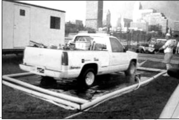
Figure P.3 Containment System Preventing Wash Water from Entering the Storm Drain.
