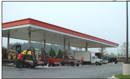
Figure 1: Covered Retail Gas Operation Without Containment for Potential
