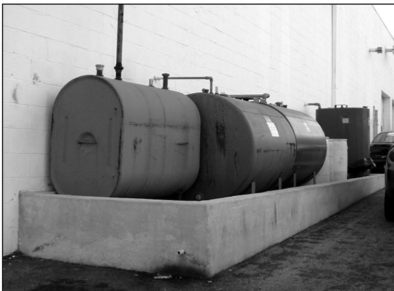
Figure P.6 Secondary Containment of Storage Drums Behind a Car Repair Shop.
