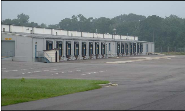
Figure P.4 Unloading Area of Warehouse.
