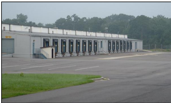
Figure 1: Loading/Unloading Area of Warehouse
