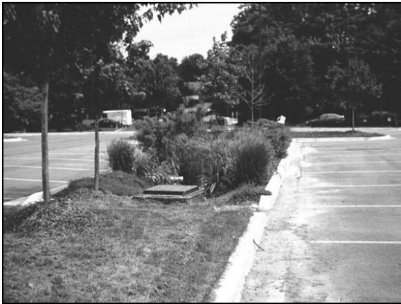
Figure 2: Parking Lot Island Turned Bioretention
