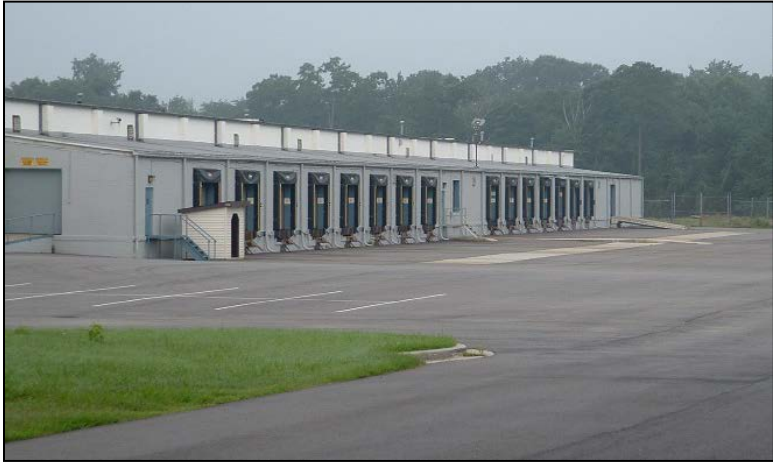
Figure P.4 Unloading Area of Warehouse.
