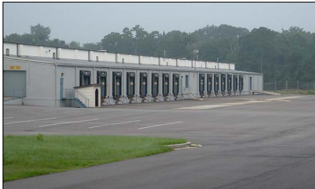
Figure P.4 Unloading Area of Warehouse.
