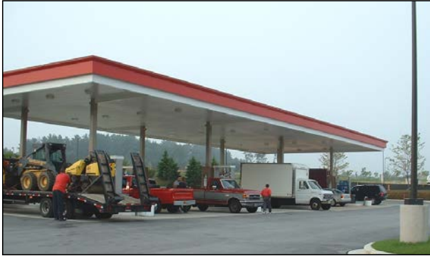
Figure PQ.2 Covered Retail Gas Operation Without Containment for Potential Spills.
